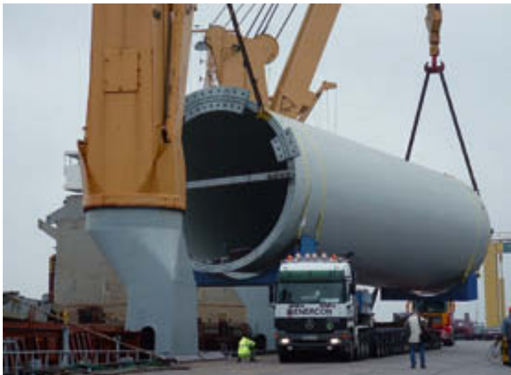
Loading one tower segment: The complete tower consists of four segments and weighs 741 tons.
