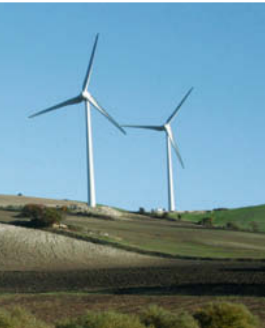
ENERCON wind turbines in San Chirico: Operators in Italy are assured dependable support and security, a fact that the Italian bank Banca Verde definitely appreciates.
